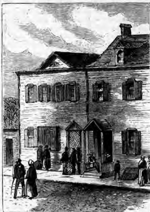
OLD POST-OFFICE IN GARDEN STREET.
