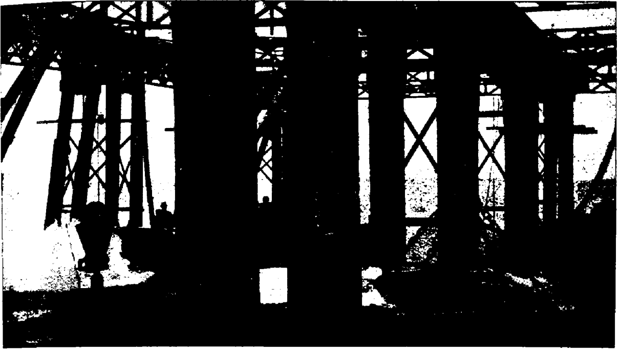
THE DIVING-BELLS USED DURING THE EXTENSION OF FOLKESTONE HARBOUR. ONE BELL JUST SUBMERGED, IS INDICATED BY THE SPLASH; THE ROOF OF THE OTHER APPEARS ABOVE THE WATER.
