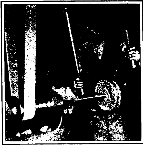
FIG. 7.—Polishing the frame on an emery wheel.
