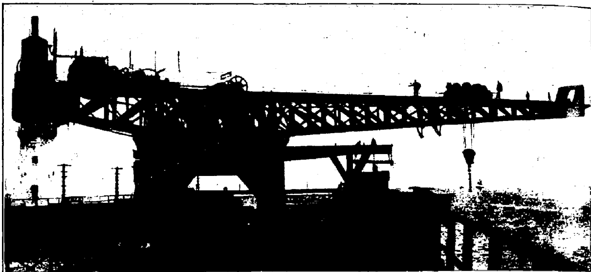
THE CRANE FOR TABLE BAY HARBOUR, TEMPORARILY IN USE AT TYNEMOUTH.
