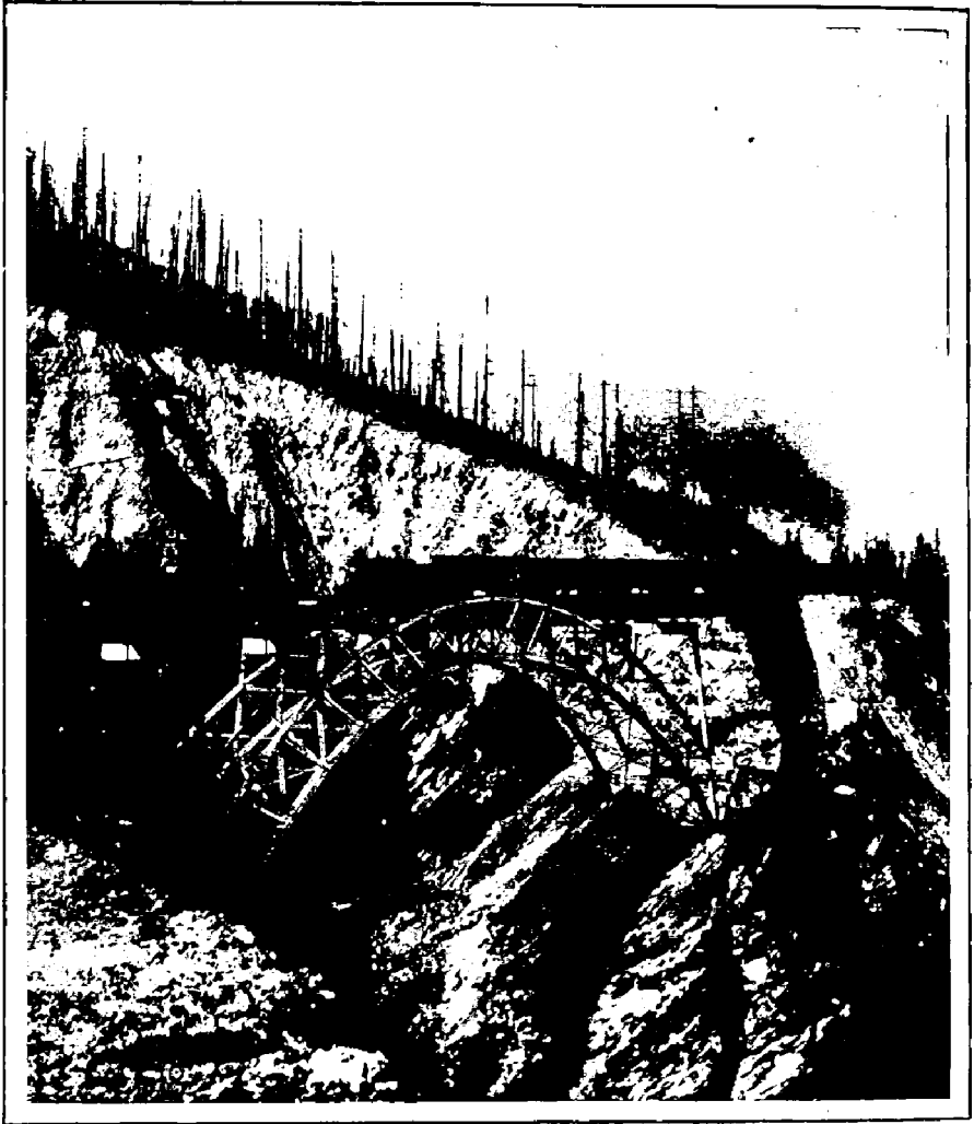
STONY CREEK BRIDGE, NEAR ROGERS PASS, B.C. A fine example of bridge construction on the C.P.R.
