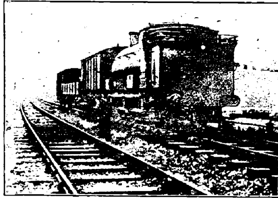
THE "P.W." TRAIN CREEPS GINGERLY OVER THE NEW LINE AS IF TO PROVE THAT THE RAIL IS WELL AND TRULY LAID.
