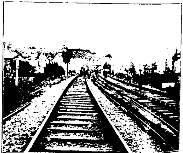
DEMOLITION COMPLETED. NEW "DOWN" TRACK BEING "TRUED," WITH OLD "BAULK" ROAD LYING LOPSY-TURVY IN THE MIDDLE
