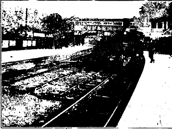
CROSS-TIES ON "DOWN" LINE LOOSENEED READY FOR DEMOLITION. NEW "CROSS-SLEEPERS" TRACK LYING MADE-UP IN THE "SIX-FOOT-WAY" READY FOR TRANSPOSITION.
