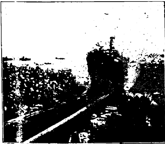
LAUNCH OF THE Meteoro , THE FIRST STEEL STEAMER BUILT IN CHILE (UNDER THE SUPERVISION OF BRITISH ENGINEERS). THE PHOTO SHOWS THE SHIP AT THE MOMENT OF TAKING THE WATER.
