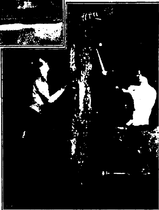
THE PICTURE BELOW SHOWS TWO MEN SETTING A PROP IN A HIGH SEAM.
