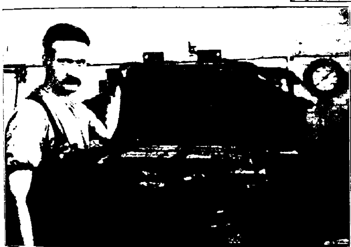
REMOVING THE WAX IMPRESSION FROM FORME ON HYDRAULIC PRESS.
