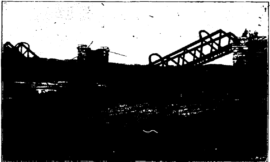
BRIDGE OVER TUGELA AT COLENBO—AFTER THE BOERS HAD BLOWN IT UP.
