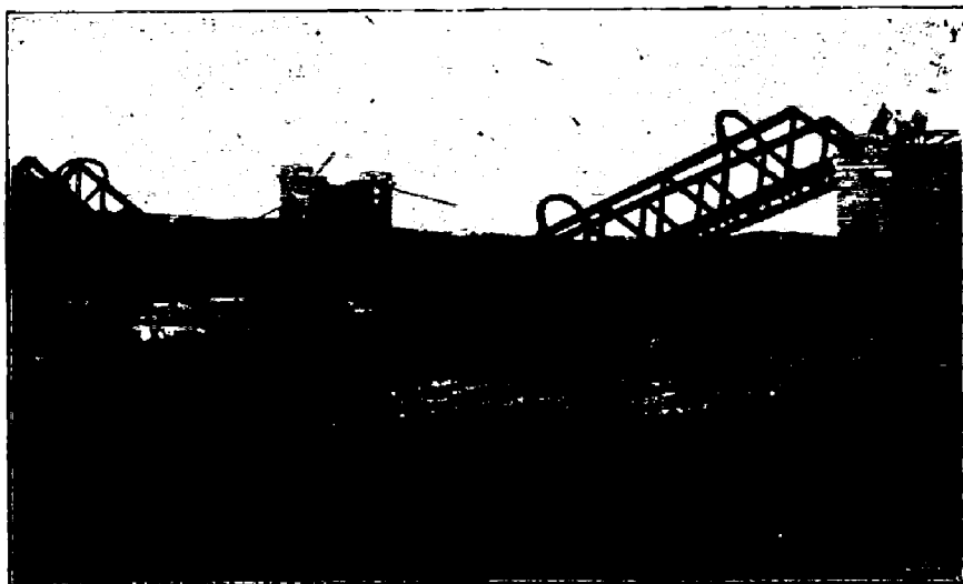
BRIDGE OVER TUGELA AT COLENSO—AFTER THE BOERS HAD BLOWN IT UP.
