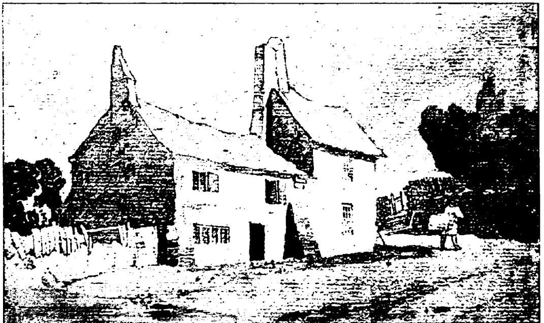
OLD HOUSES, MILL LANE
