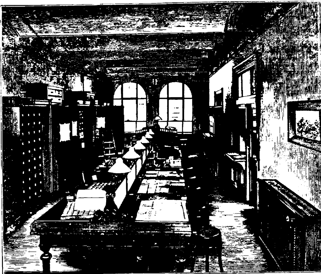
INSIDE VIEW OF PREMISES.
