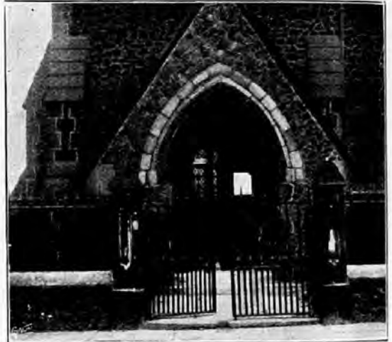
THE PORCH OF THE "SLAG CHURCH," HOLY TRINITY.
