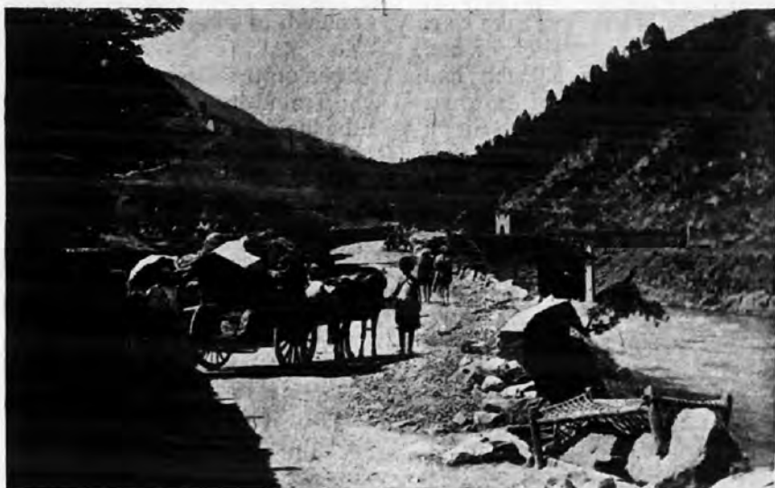
BRIDGE AT KOHALA.
