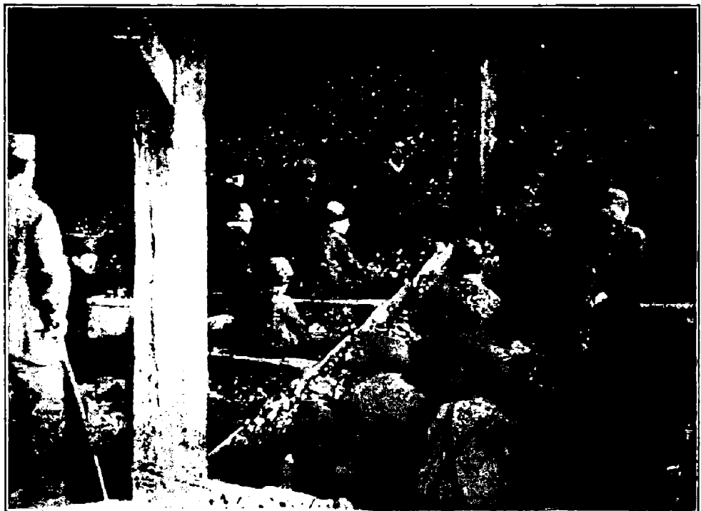
THE CHUTES WHERE THE BREAKER BOYS PICK SLATE FROM THE COAL.
