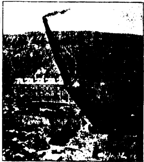
Felling a 200-Foot Stack.
