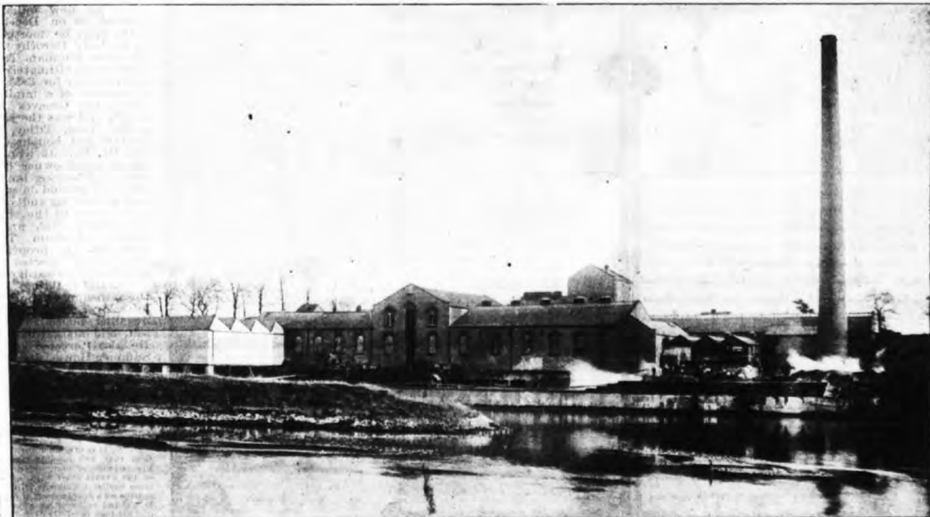
General View of Mill Bank Paper Mill.
