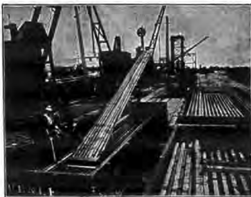
Unloading Steel Rails from Cars to Vessels at Lake Port.
