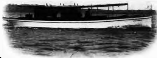
42-ft. x 14-ins. draft Launch for the Amazon, speed 12 miles.
