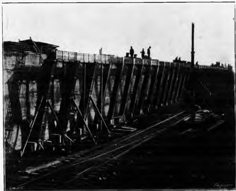
NEWPORT DOCK.—CRANE ROAD. MOULDS FOR FERRO-CONCRETE STRUTS ( see page 329 ).
