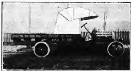
30 H.P. Type "D" 4 Cylinder 2 Ton Lorry.
