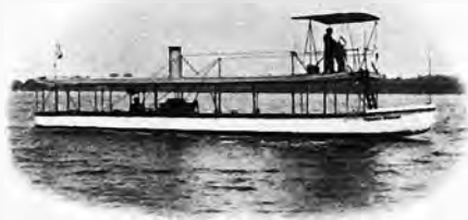
65 ft. Motor Canoe, 14 in. draft, for Pahang River, Straits Settlements.
