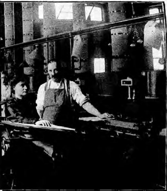
Inserting sheets in the gumming machines.
