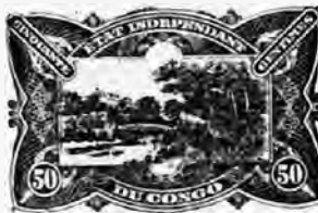
(Railway bridge over the M'pozo.)
