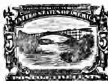
(Bridge at Niagara Falls.) 86
