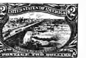
(Bridge over Mississippi at St. Louis.)
