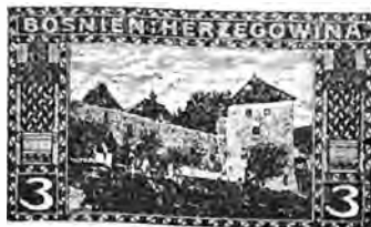
(Plima Tower at Jaice.)
