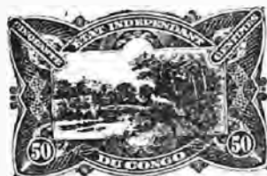
(Railway bridge over the M'pozo.)
